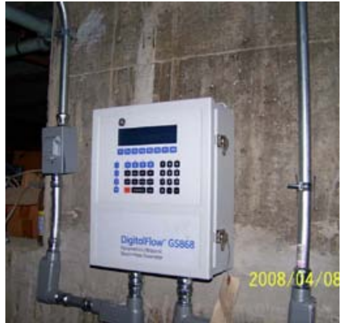
GS868 Flow Computer Transit-time ultrasonic meter
